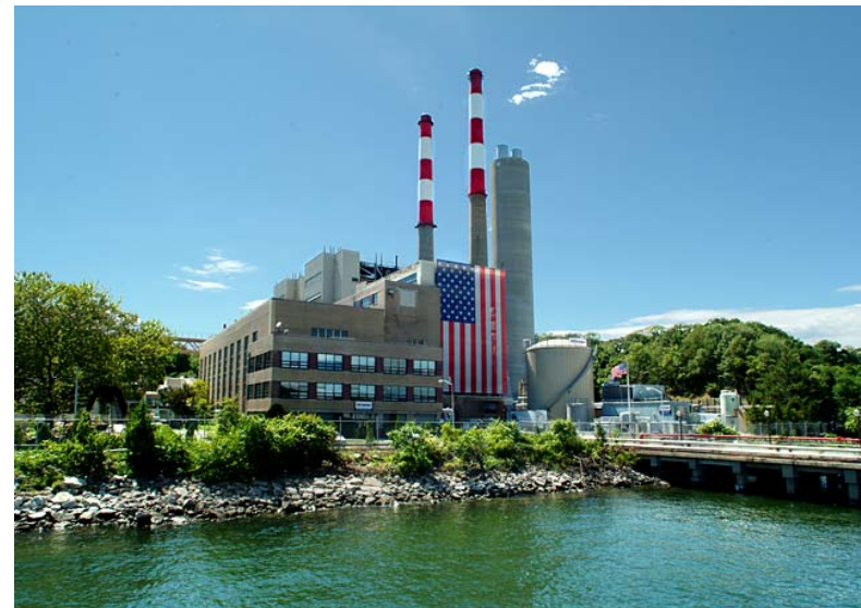
Port Jefferson 450 MW
